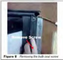
Figure 8 Removing the bulk seal screw
